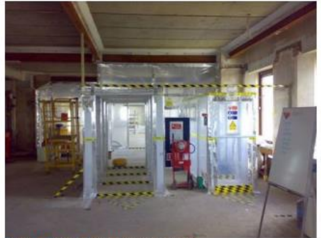
Figure 3 – Typical asbestos removal enclosure
