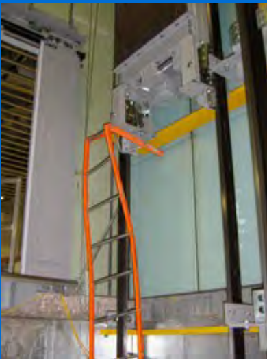
The ladder from which Kevin Dawson was working when he was struck and killed by the heavy counterweight.
